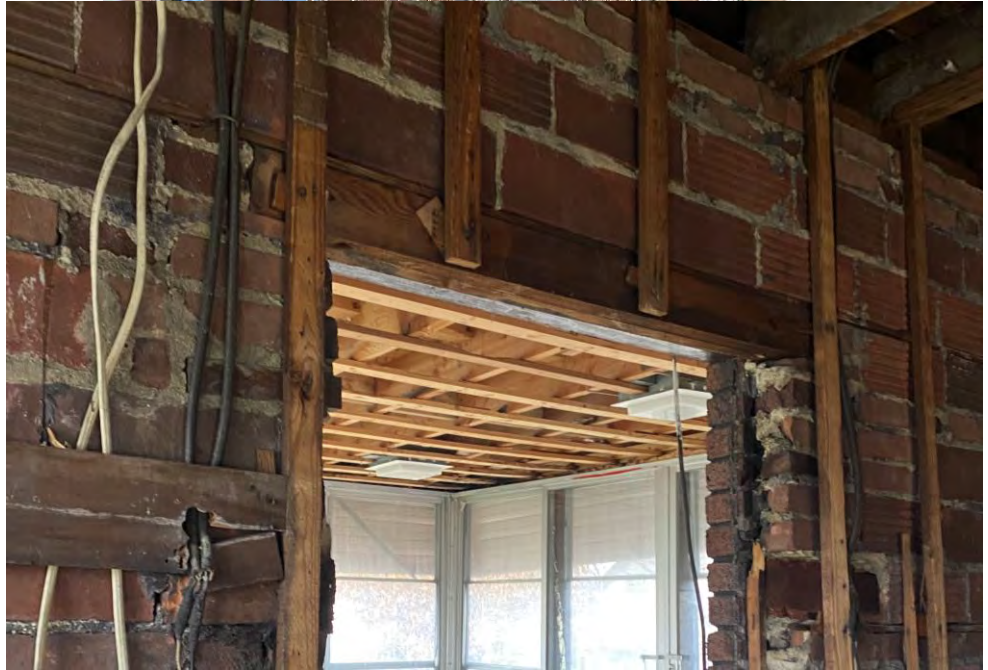
2ND FLOOR PORCH CEILING/ROOF FRAMING
