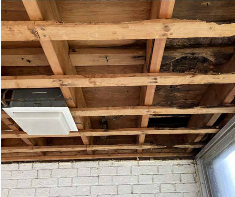
2ND FLOOR PORCH CEILING/ROOF FRAMING
