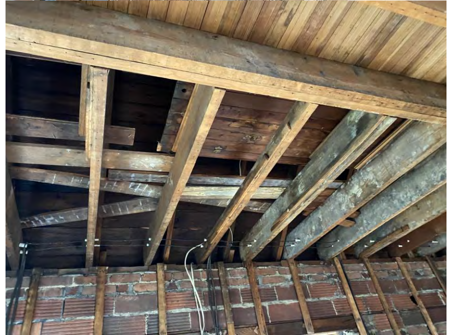
ORIGINAL ROOF FRAMING
