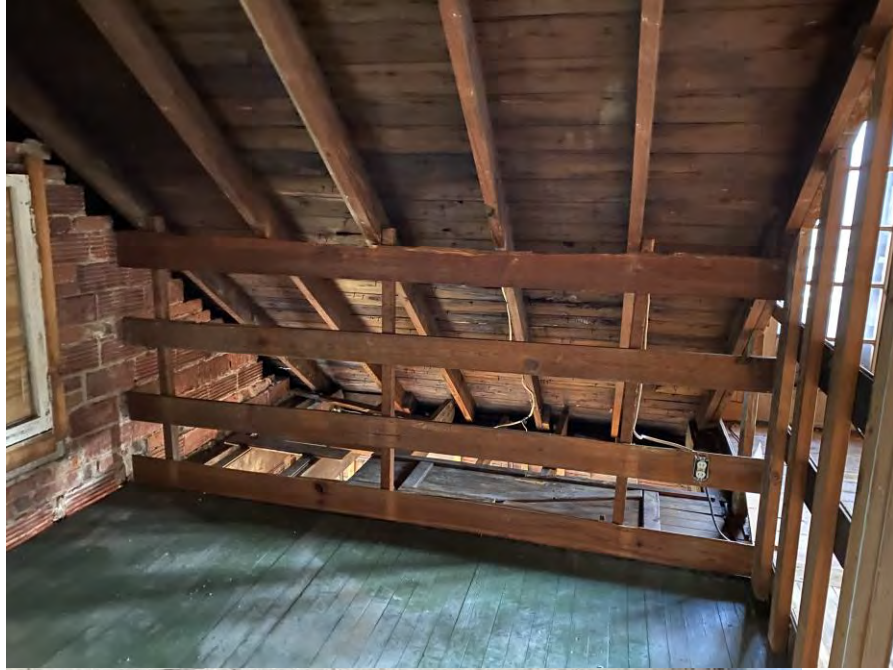
ORIGINAL ROOF FRAMING
