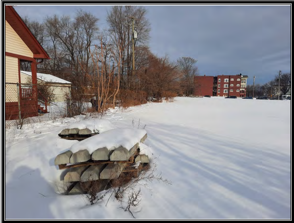
Photo 3: Viewing at construction materials observed on the southern portion of the property.
