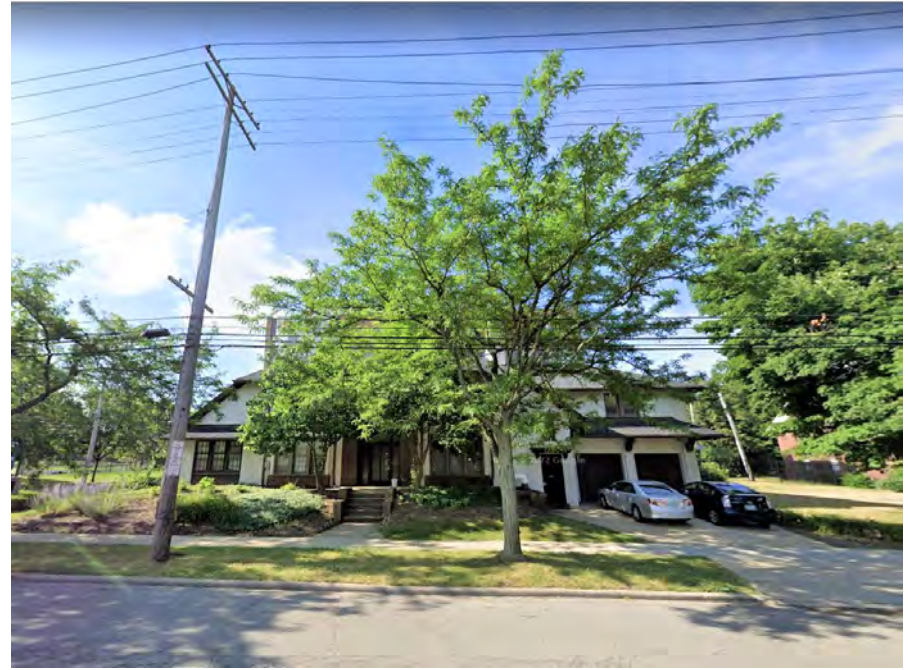
CWRU SUSTAINABILITY HOUSE & STJ RESIDENCE HALL
