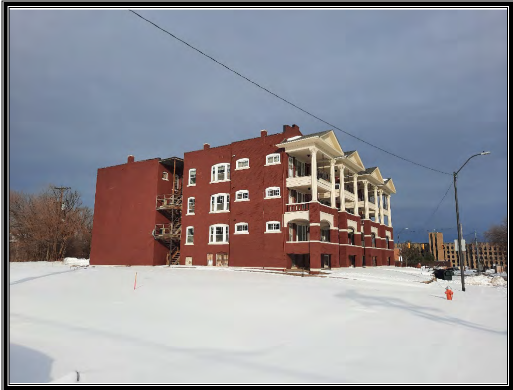
Photo 7: Viewing at the north adjoining multi-tenant residential building.
