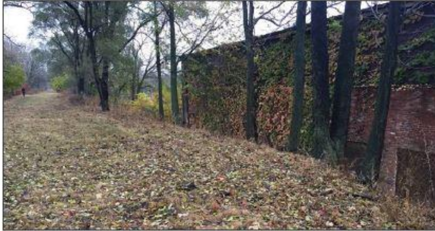
At Ashland Ave looking East
