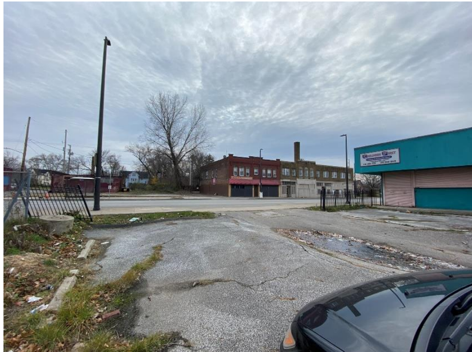
PARKING LOT – CURRENT CONDITIONS
