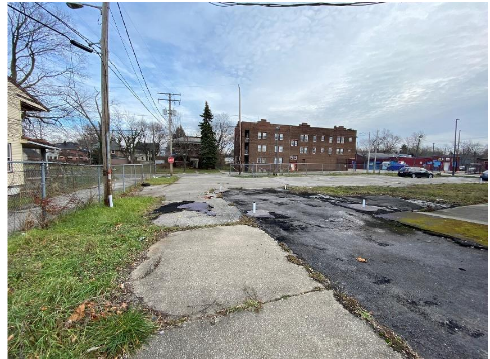
PARKING LOT – CURRENT CONDITIONS
