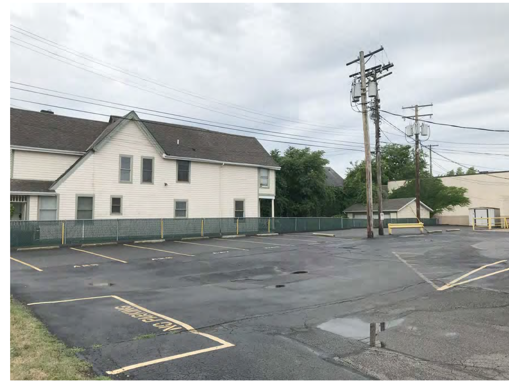
VIEW OF NORTH SIDE OF SITE FROM 48TH STREET - ACROSS EXISTING COMMERCIAL PARKING LOT 4 IMAGE OF EXISTING A001 NO SCALE
