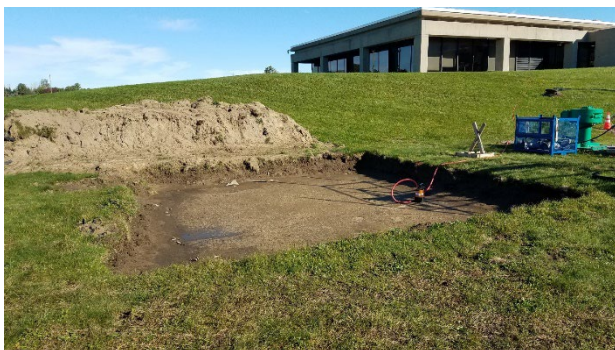
Lake Huron WTP reservoir access hatch BEFORE
