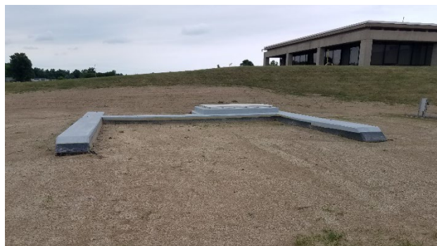
Lake Huron WTP reservoir access hatch AFTER
